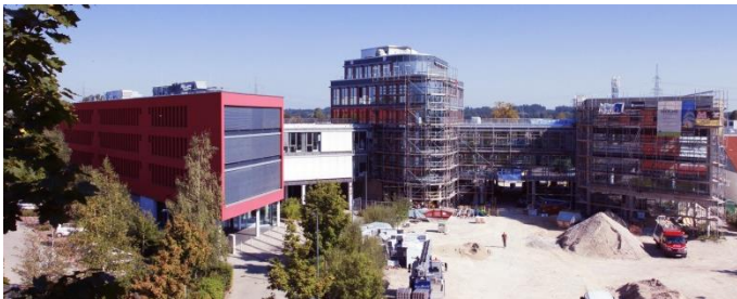
Headquarters of Scanlab GmbH © Scanlab
